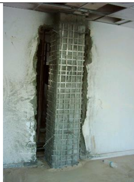
Fig. 5 Grouting and zinc mesh installation
